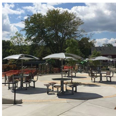
Construction progress at Settlers Grove Riverside Park Photo courtesy of Ada Village
