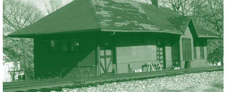
Once Upon a Time Ada had a train depot! This photo from 1979 depicts the Grand Trunk Western Railway depot after its years of service. The depot stood between Bronson St. and the railroad tracks just before the intersection with Headley St. This was a very active spot for a hundred years from the arrival of the first locomotives in the 1850s. Sadly, the building was torn down in 1986. The ADA shingle that hung out along the platform is on display at the Museum.
