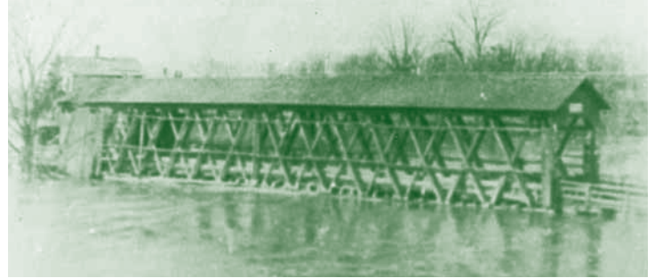
Deep and Wide. 1904 and 1905 also brought record flooding to Ada. The covered bridge was in danger of being swept away. Several measures were taken for its protection. Farmers parked wagons loaded with rocks on the bridge to weigh it down. The boards were removed from the sides to allow water to flow through the bridge. The bridge was even secured with a big cable to a nearby elm tree.
